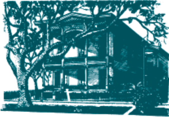
Rudolph Kruger House, 1628 Postoffice
